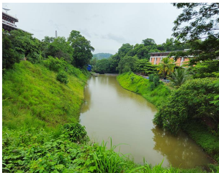
Rainwater Harvesting Pond-2
